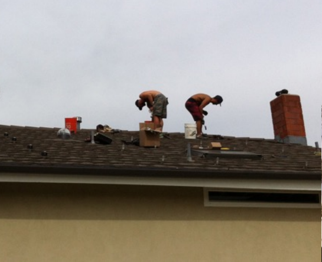
Installing Brackets Under Shingles
